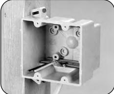
2. Insert the conductors from the outside of the box into the appropriate knockout and OVER **THE TOP** of the Speed "K" Klamp until the outer jacket extends at least 1/2" past the top of the clamp.
