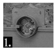
Mount electrical box to exterior wall and feed wiring through knockout prior to siding.
