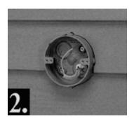
Affix mounting brackets, and caulk around box after siding is installed.
